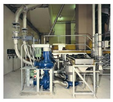
In addition to the gentle handling requirements at the start of raw produce processing, the Hidrostal range is also suited to the energy efficient circulation and removal of the washwater used to clean raw produce. This often contains grit, sand, peelings and vegetable lumps.
